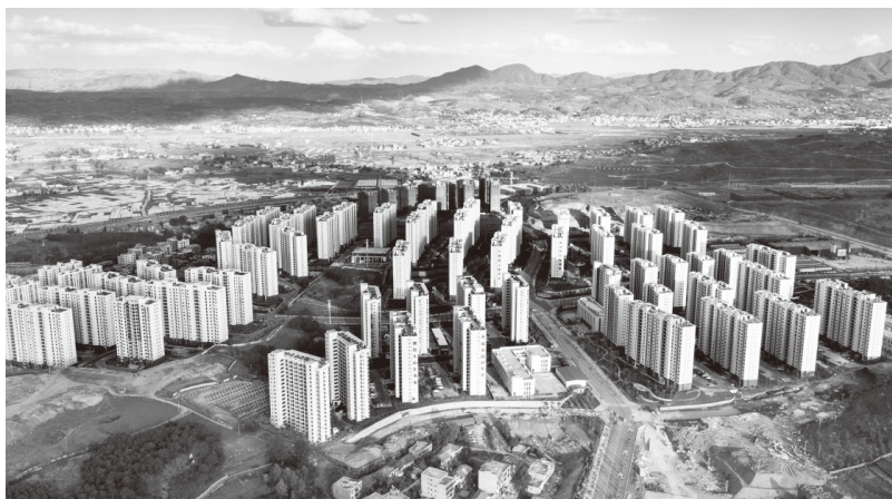
▲鲁甸县卯家湾易地扶贫搬迁安置区全貌
